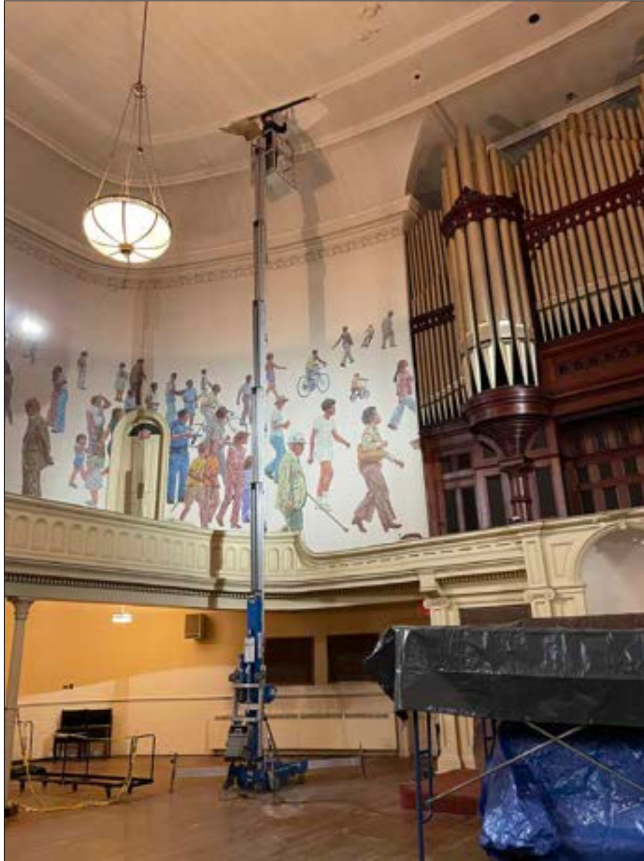
Photo 02. Detail of personnel lift allowing direct access for hands-on inspection.
