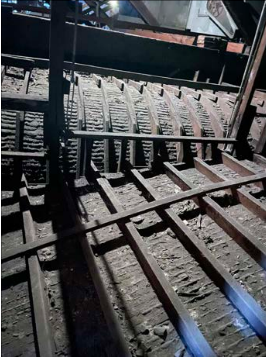
Photo 06. The quality of keying within the covered cornice is clear; its geometry helps to sustain its formidable condition.
